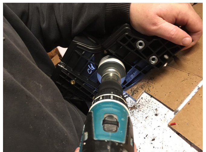
Use 2 3/8" hole saw, same as 60mm. Run blade in reverse. Drill holes.
