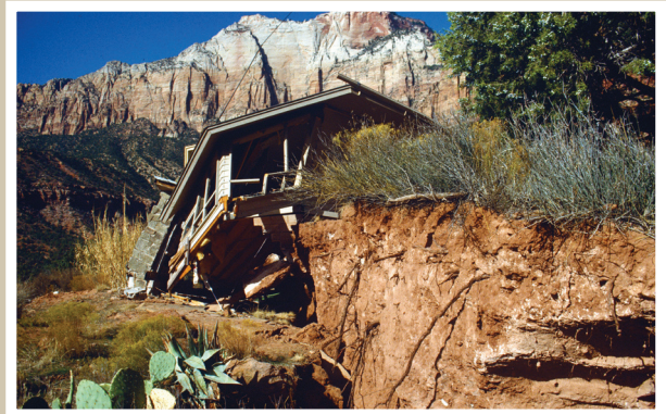
Home destroyed by the Springdale landslide, triggered by the September 2, 1992, M 5.5 St. George earthquake. Photo courtesy of the Utah Geological Survey.
