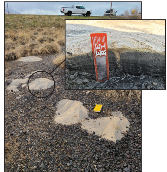
Sand boils near the Great Saltair event center caused by ground-shaking-induced liquefaction from the Magna earthquake. Photo courtesy of the Utah Geological Survey.
