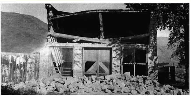
Damage caused by the M 5.5 Elsinore, Utah, earthquake of 1921 (above) and by the M 5.8 Richmond (Cache Valley) earthquake of 1962 (right). (Photos courtesy of, respectively, the F. J. Pack Collection, Special Collections Department, University of Utah Libraries, and Ariel D. Benson, Richmond, Utah)
