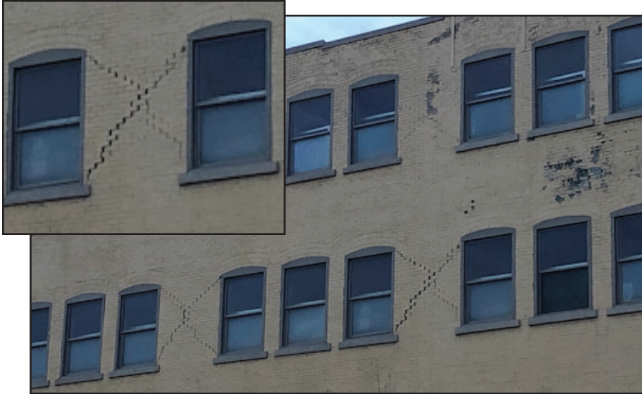
Damage to a URM building in downtown Salt Lake City from the 2020 Magna earthquake. The "X" pattern between the arched windows is a telltale sign of URM construction. This is an example of "in-plane" failure. Photo courtesy of Reaveley Engineers.
