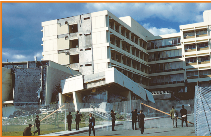
This hospital in Sylmar, California, had to be demolished after the 1971 M 6.7 San Fernando earthquake. Photo courtesy of the U.S. Geological Survey.
