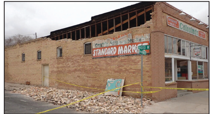
Structural damage to an unreinforced masonry building in downtown Magna caused by strong ground shaking from the Magna earthquake. Photo courtesy of the Utah Geological Survey.
