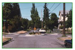
This traffic calming device is a circular island that is generally placed at intersections around which traffic flows in a counterclockwise direction. This device has the potential to reduce speed and accident severity and improve capacity. Some of the negative aspects of traffic circles are driver unfamiliarity (yielding to the vehicle on the left), and vehicles may encroach on pedestrian crosswalks and bicycle travel lanes.
