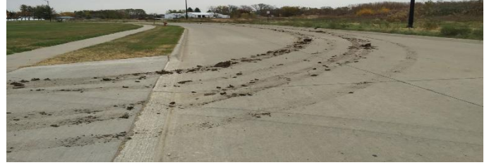
Track mud into the roadway
