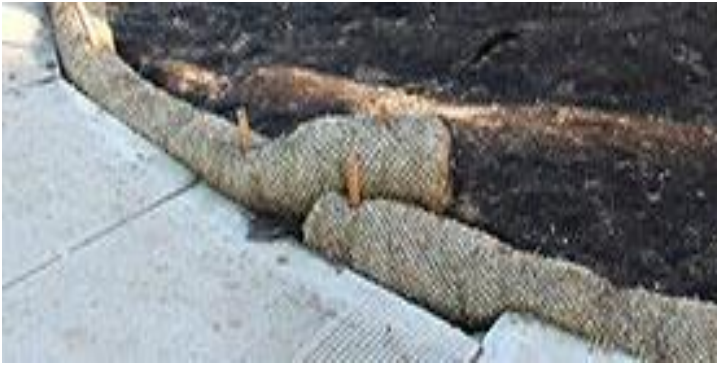
Straw waddles help with sediment control
