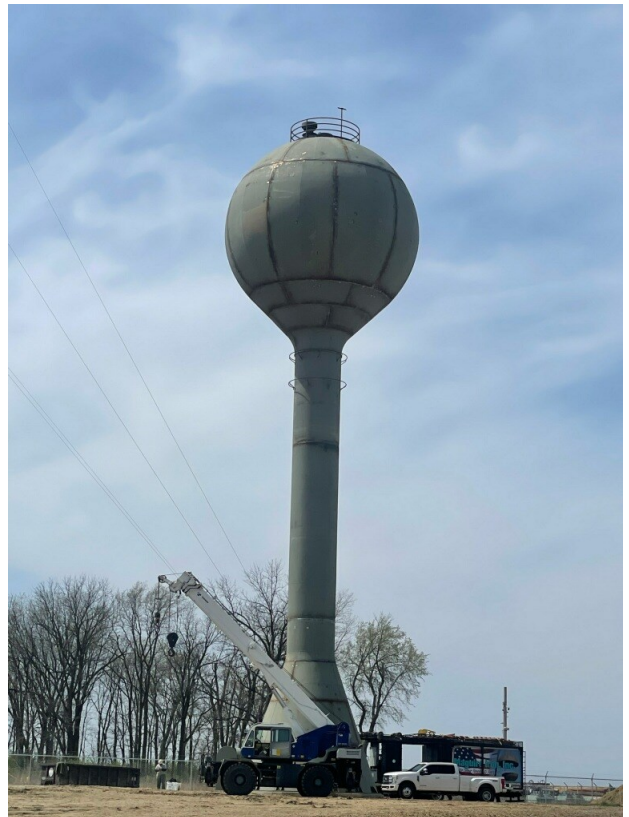
Downs Crossing Water Tower completed April 11
