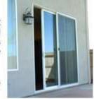
The two main vulnerabilities of the door are that it may lifted out of its track and that it may be forced to slide open. Let's first deal with coming out of the track...
