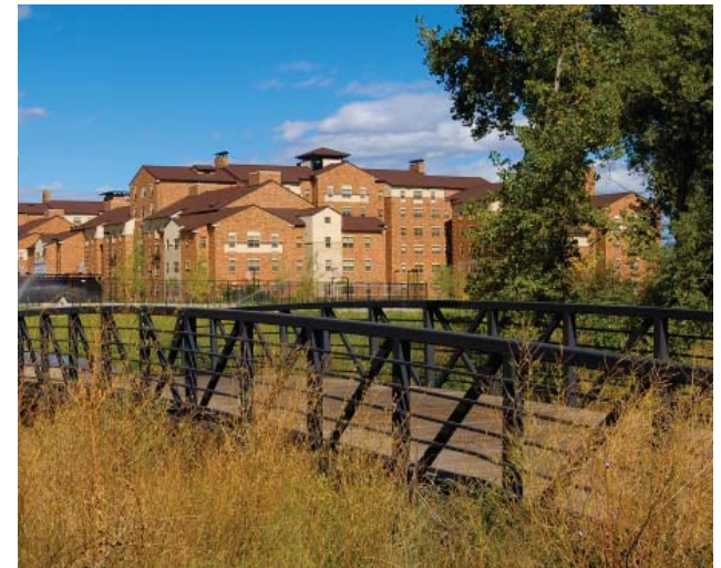
Connections to the wetland landscape should be provided from the auto-oriented district of the West Forest Street area.
