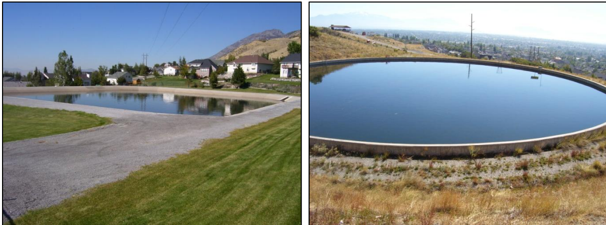
Shown above: Secondary water reservoirs that are part of the pressurized irrigation system.
