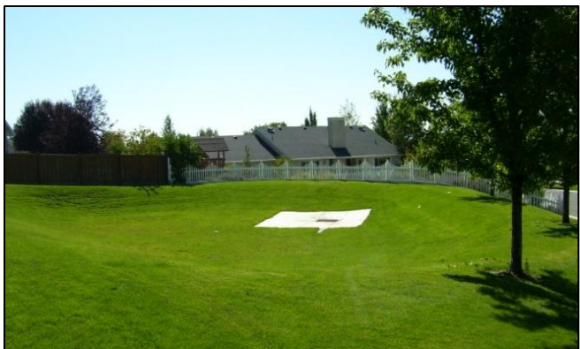
A storm water detention basin maintained by Lindon City. Many basins serve dual functions as both public park green space and storm water control. (2009)
